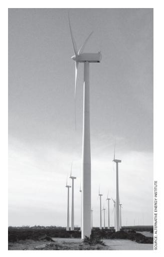
**LARGE MODERN WIND TURBINES** In foreground is the 1.65 MW wind turbine at Big Spring; in the background are 660 kW units.
