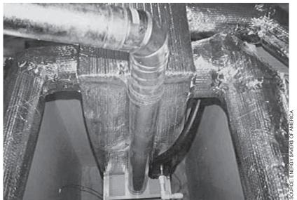
**ATTIC DUCT SYSTEM** Insulating and sealing ducts can be one of the most cost effective ways to save energy.
