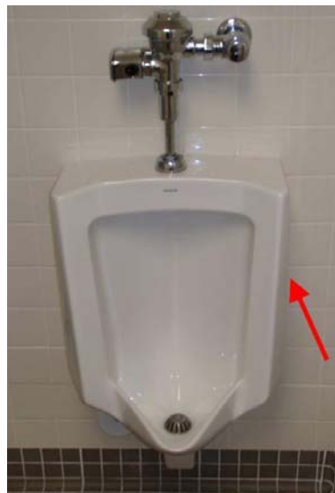
The gallons per flush (GPF) used by a urinal may be indicated on the side of the fixture.
