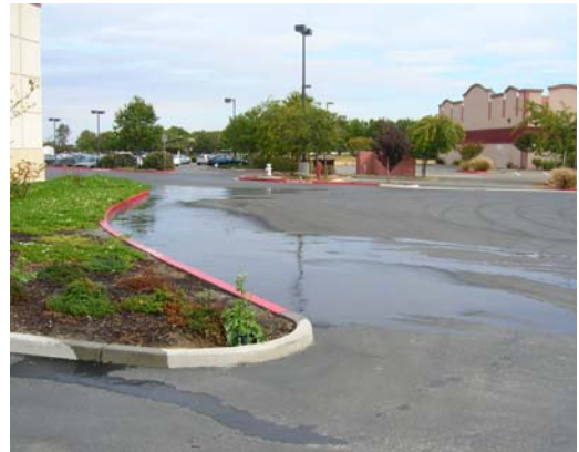
Often, landscape irrigation runs off into parking lots or other paved areas.
