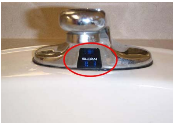
If a faucet has a motion sensor, it is located near the base of the fixture.
