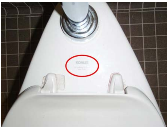
The gallons per flush (GPF) used by a toilet is usually indicated near the rear of the fixture.
